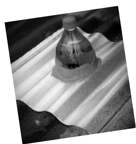
Place the solar bottle bulb into the hole.
