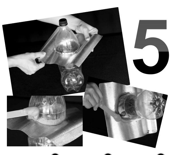
Insert the bottle into the GI sheet until the upper third. Apply rubber sealant on the strips above and around the area below.
